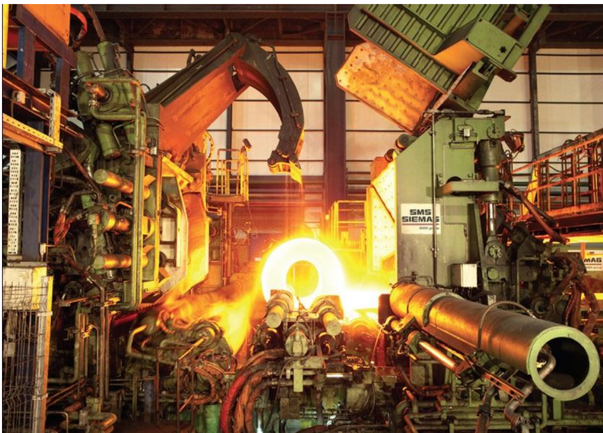
Fig. 1. "Coilbox" of the compact hot strip mill (Çolakoglu Metalurji AS, Turkey)
